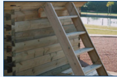
Wooden external stairs in treated red pinewood
